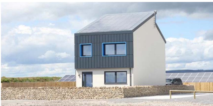
SOLCER house. Source: Cardiff University
